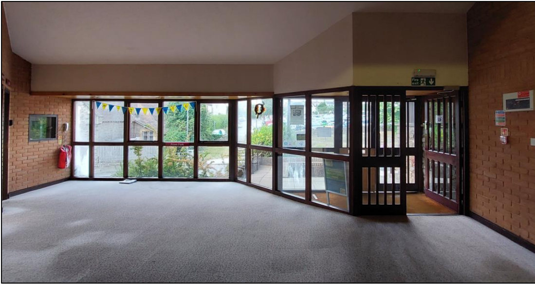
Existing foyer entrance.
