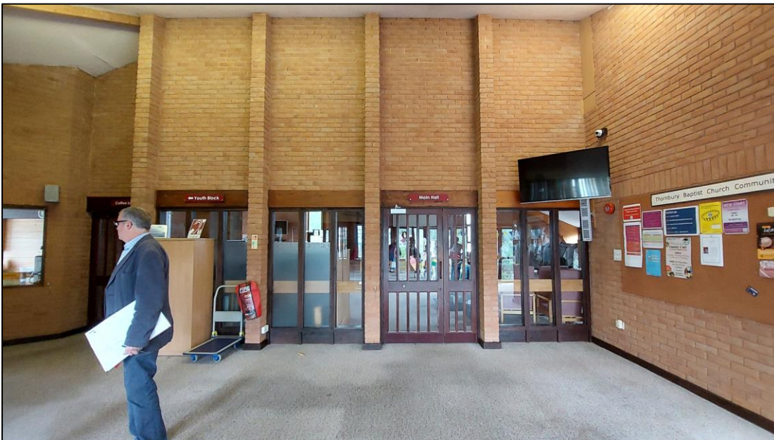
Existing doors leading to the auditorium.
